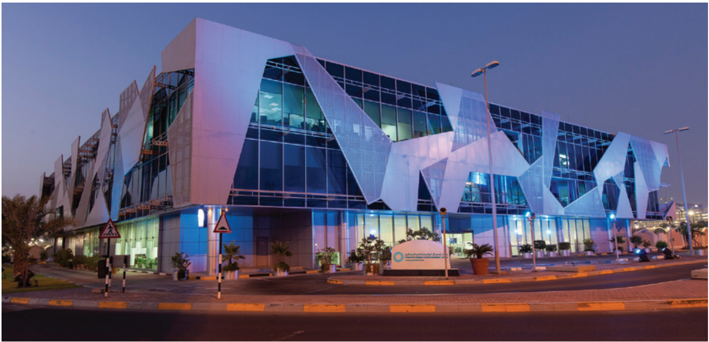
The state-of-the-art diabetes facility in Al Dhafra, set to open later this year.
