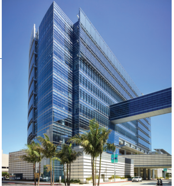
Cedars-Sinai Pavilion Building
