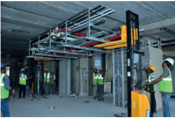
Meitra modular hospital under construction
