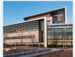
Spaulding Rehabilitation #6 in Rehabilitation
