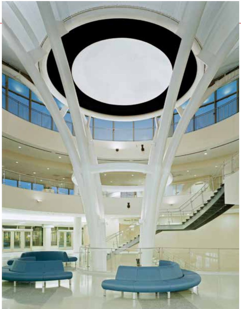
This connection between nature and healing continues on the interior of the hospital, starting at the lake-level entry. A stunning, four-story atrium features a 21-meter-diameter central support nicknamed the “Tree of Life,” its eight structural columns curving outward and upward like tree limbs.
