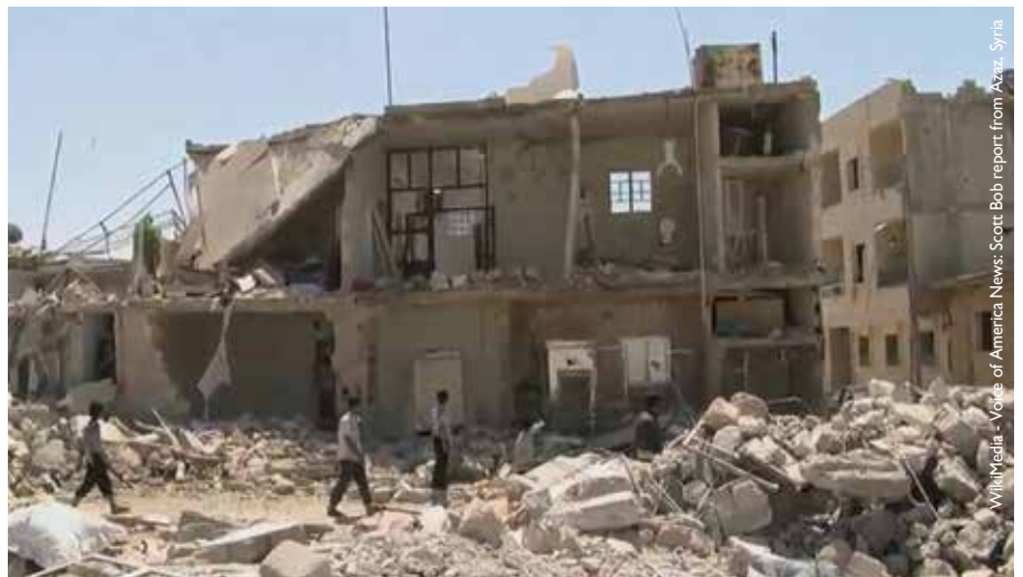
Bombed buildings in Azaz, Syria. 16 August 2012
